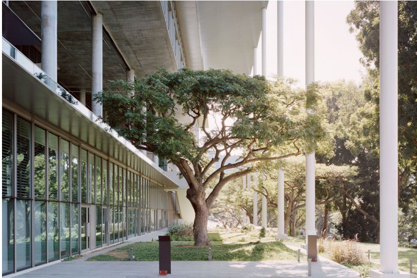
NUS SDE4, Singapore's First New-Build Net-Zero Energy Building
