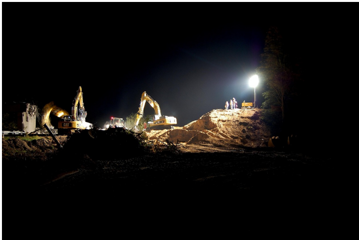
Figure 1: Construction Activities at Night: An Illustration
